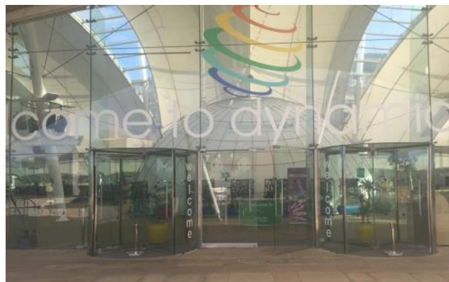
Main Entrance of Dynamic Earth showing double glass pull and two revolving door.
