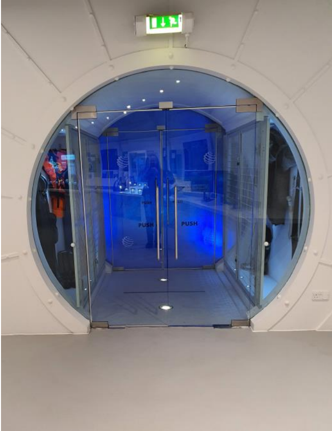
Left: Exit from 'Discover the Deep' into Polar Extremes. This is a double set of double-doors. Each set is a push door.
