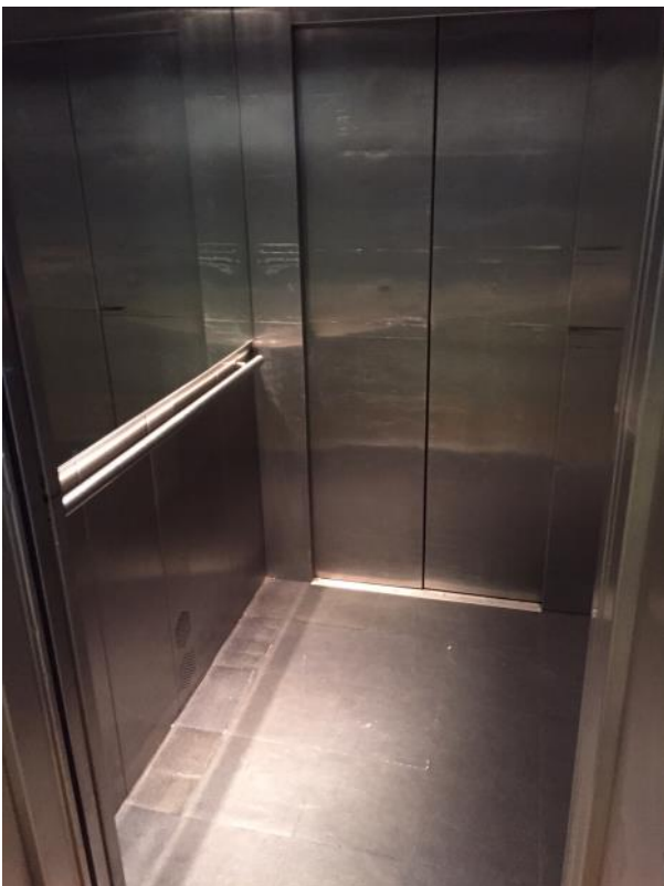
East side lift.
